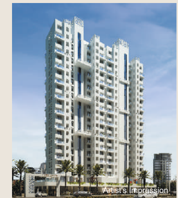
ONGOING PARTH SKYONE DOMBIVLI - EAST
