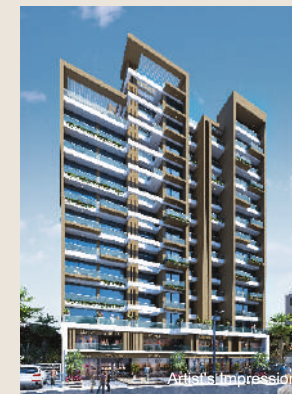
COMPLETED PARTH MAGNUS SANPADA, NAVI MUMBAI
